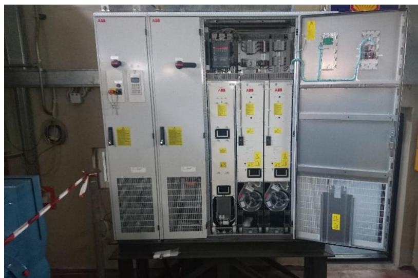
Fig. 8. The cabinets that host the electrical drives for the dynamometer and motor/generator.
