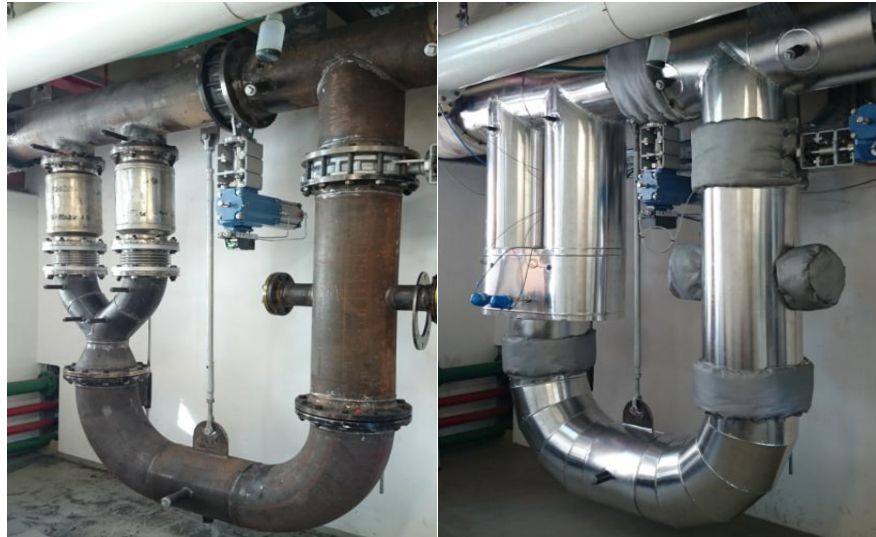
Exhaust Bypass System, CAT3176B
